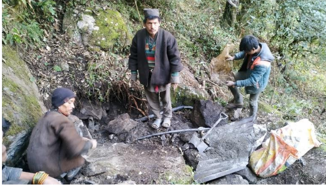
Under construction of intake for h5,h6 and h8
